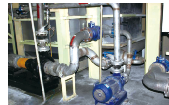
水洗工位增加喷淋系统 Spray system with water washing station
